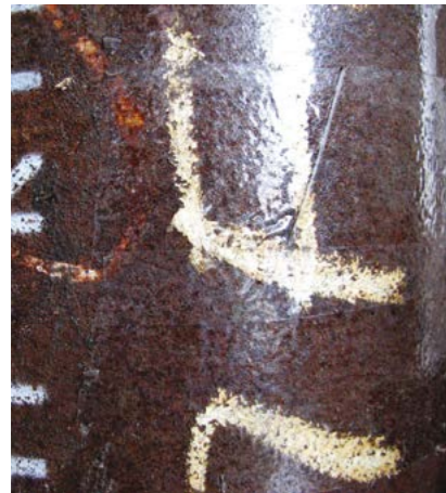
API 5L Piping
