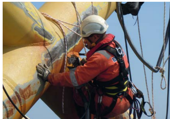
Bristle blaster® on an offshore platform
